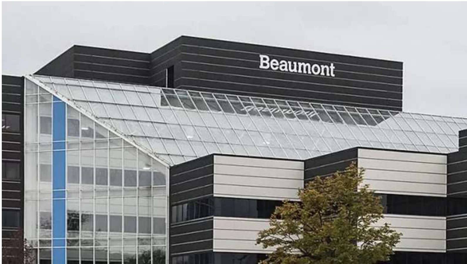
Beaumont Service Center, Southfield
